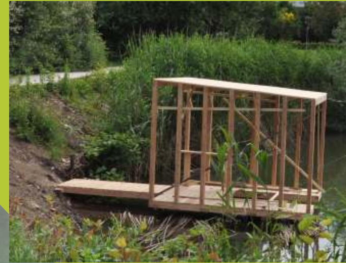
A dock at Koseze pond during construction.
